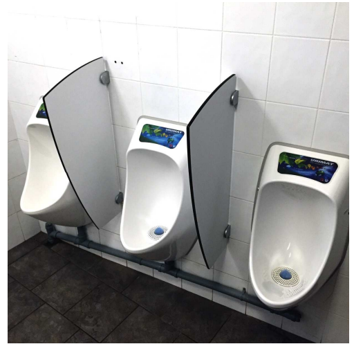
Unconcealed waste-pipe visible below the urinal
