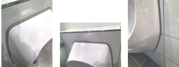
Please ensure that the urinal and wall-junction-seal are mounted firmly against the wall. This not only provides stability to the whole unit (in case of vandalism) but also deters easy removal of the walljunction-seal, which generally happens where it is just hanging off the urinal.
