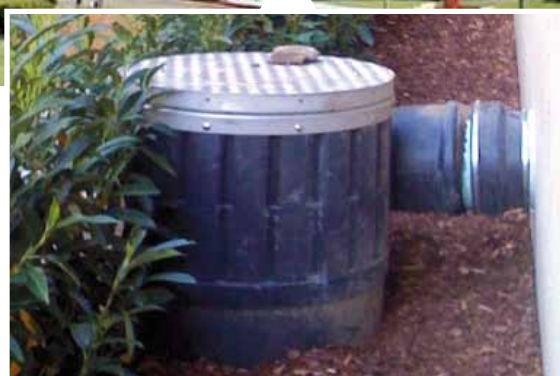
The WFF 300 vortex fine filter. The rainwater flows into the filter unit through an above ground pipe that exits directly from the building wall. The outlets for the filtered water and the residual dirty water are installed below ground.
