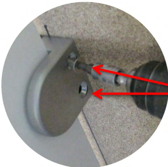
Now connect the brackets by using the countersunk head screw
